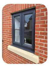
To achieve the decibel reduction rating of 43RW, an acoustic sealed unit configuration comprising Soft Coat Low-E & 10.8mm Acoustic Laminated Glass was required. This added significant weight to the sashes, therefore requiring extra heavy duty hinges to be included.
